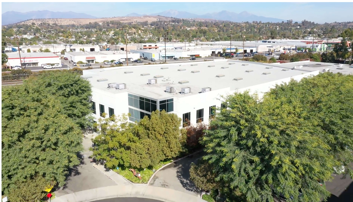
DKA Aerospace's California distribution facility in City of Industry
