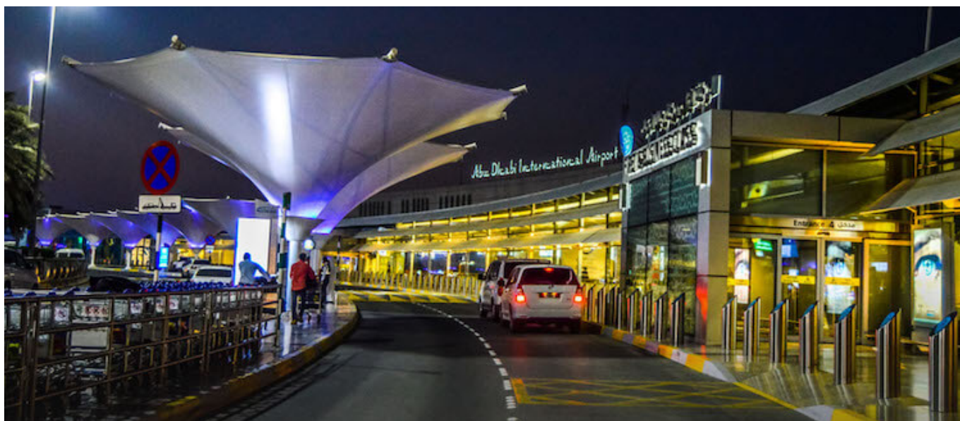
Abu Dhabi International Airport
